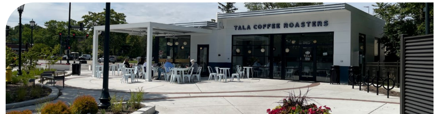
The image above shows an adaptive reuse of a former gas station into a coffee shop. Previous space used for gas pumps and cars is now dedicated to outdoor dining and flexible space that can be used for larger community events. Streetscape enhancements beautify the adjacent roadway.
