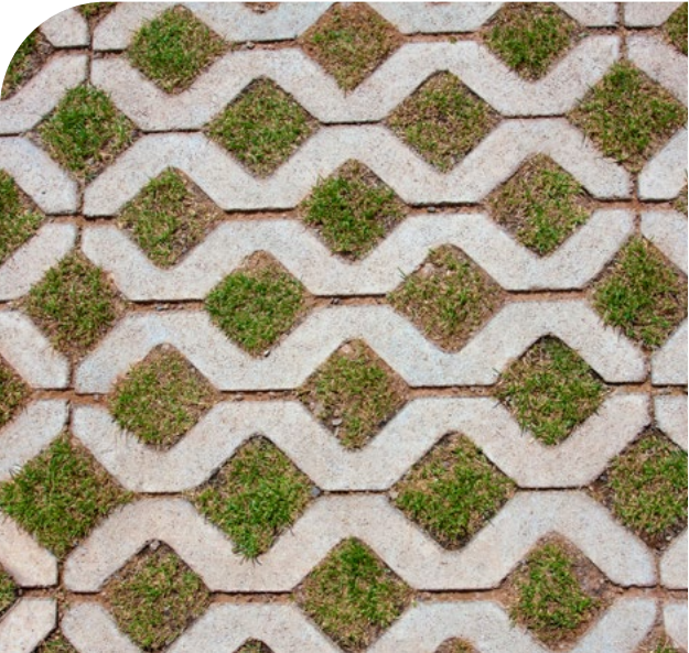
Permeable pavement helps reduce flooding, manage stormwater, and improve water quality.
