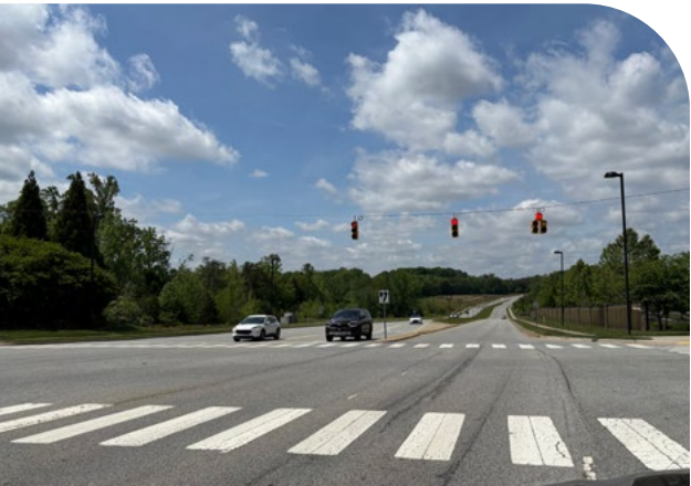
Roadways like Kernersville Medical Parkway help to close the gap in connectivity.
