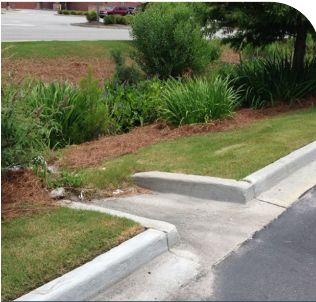
A bioswale in a Savannah, GA parking lot effectively slows, captures, and treats stormwater runoff.
